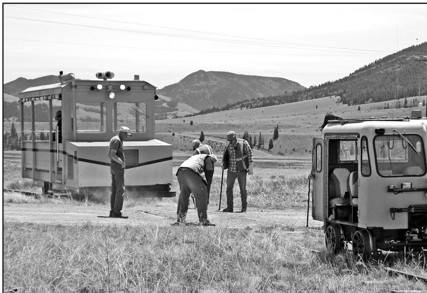
Cleaning the flangeways at a crossing with the Silver Streak waiting to cross at left. – Photo © 2013 Pat Mauro.
